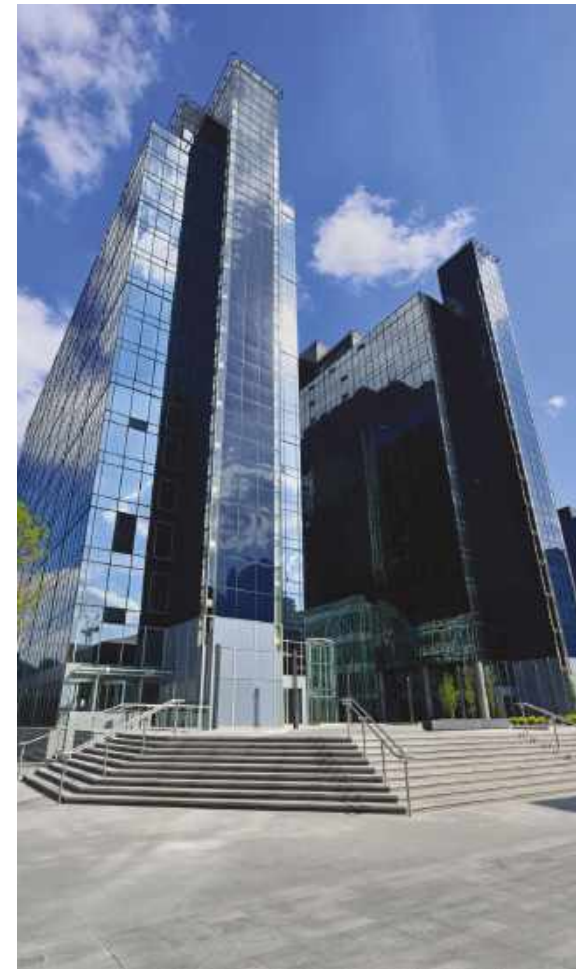
HARBOUR EXCHANGE London, UK
